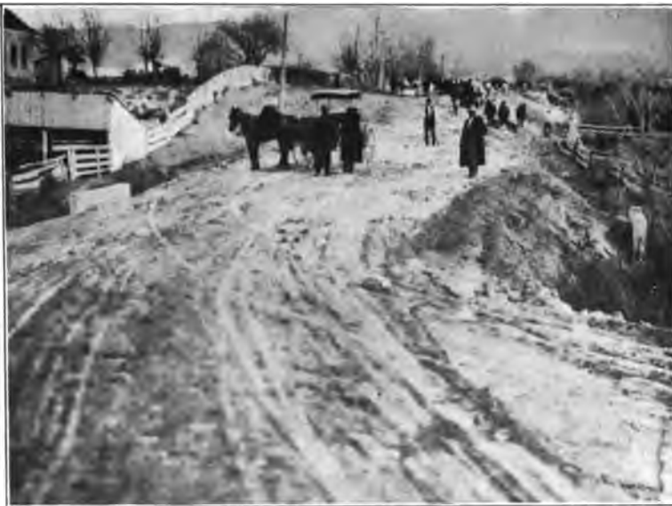
FIG. 12. CONCRETE CULVERT NEAR SPRING CITY. CITIZENS CONTRIBUTED HALF THE COST OF DOING THE WORK, WHICH INCLUDED MAKING THE DEEP CUT AND A CORRESPONDINGLY HIGH FILL OVER THE CULVERT
